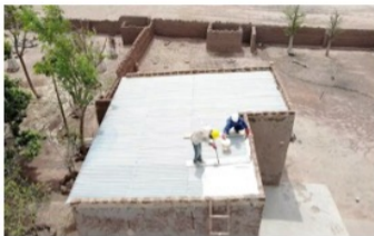
Application of cool roof coating
