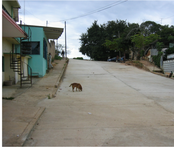
(b) After Pavement
