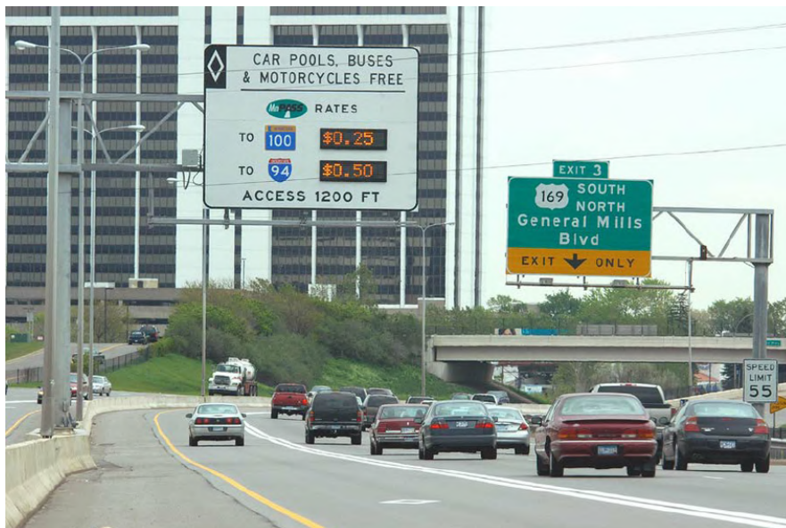
Figure 1: Snapshot of highway I-394, Eastbound direction, just before the exit to General Mills Boulevard. The Express Lane is the leftmost lane, separated by the rest of the highway by a double white line on the ground. Source: Buckeye (2012).
